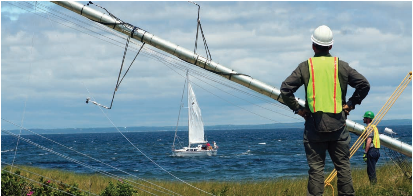
Deepwater Wind installed a temporary meteorological mast near Great Salt Pond on Block Island, R.I., as part of its comprehensive wind-resources study of the area of its proposed offshore wind farm. Photo Courtesy of Deepwater Wind
